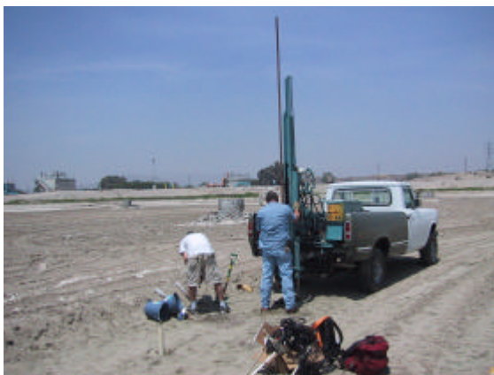
Core drilling for soil samples
