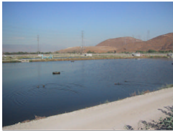
Full rapid infiltration basin, San Bernardino, CA.
