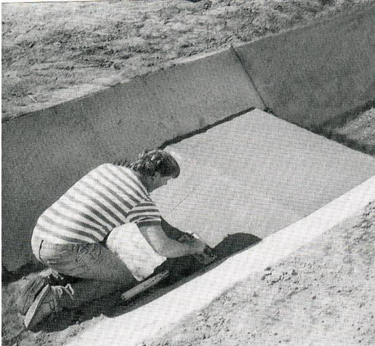
**Long-throated flumes that measure channel discharges with minimum head loss are most economical, perform with high accuracy and do not need any calibration (Replogle, 1975; Bos et al., 1984; Clements, 2001).**
